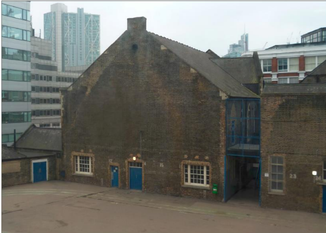
Existing courtyard elevation of Tabernacle Building
